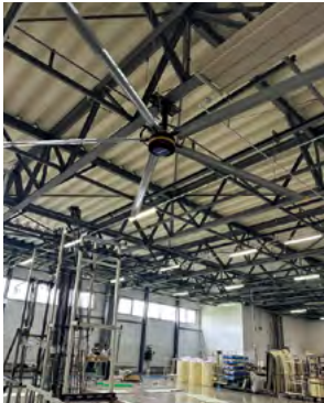
Large energy-saving fans (Gotemba Plant)
